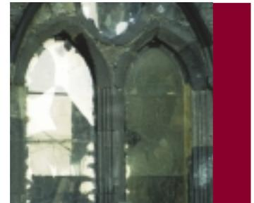
*Thin polycarbonate sheeting has been used here, giving hideous “hall-of-mirrors” distortions. This can be overcome by using 6mm thick sheet, but the reflections, whilst not being distorted, will still give the building a “blind” appearance.*
