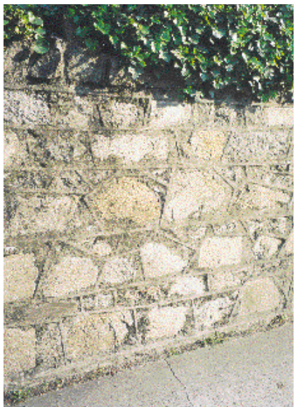
Example of crude pointing
