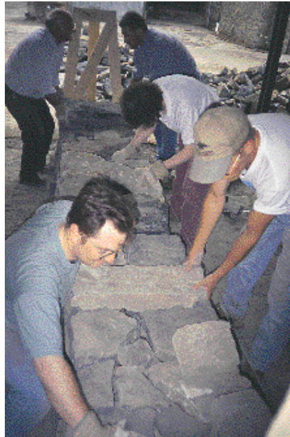
Laying through stone in double dry stone wall
