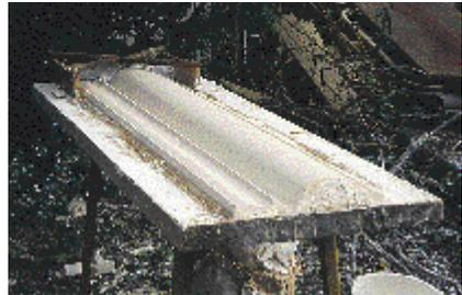
*Reverse mould showing template and horse in position.*
