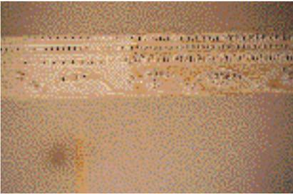
*Cleaned cornice on left contrasting with portion on right, which is obscured by layers of paint.*
